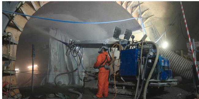
Fig. 1: Shotcrete application in a freshly excavated tunnel using a 5-DoF concrete spraying unit. Image provided by Costain Laing O'Rourke Joint Venture.
